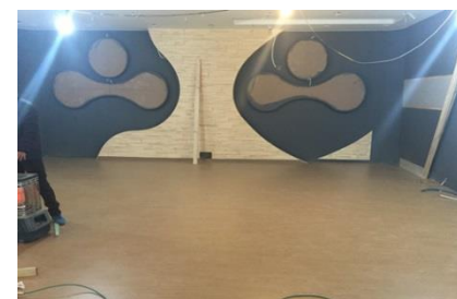
< Performance Stage – Under Construction >
